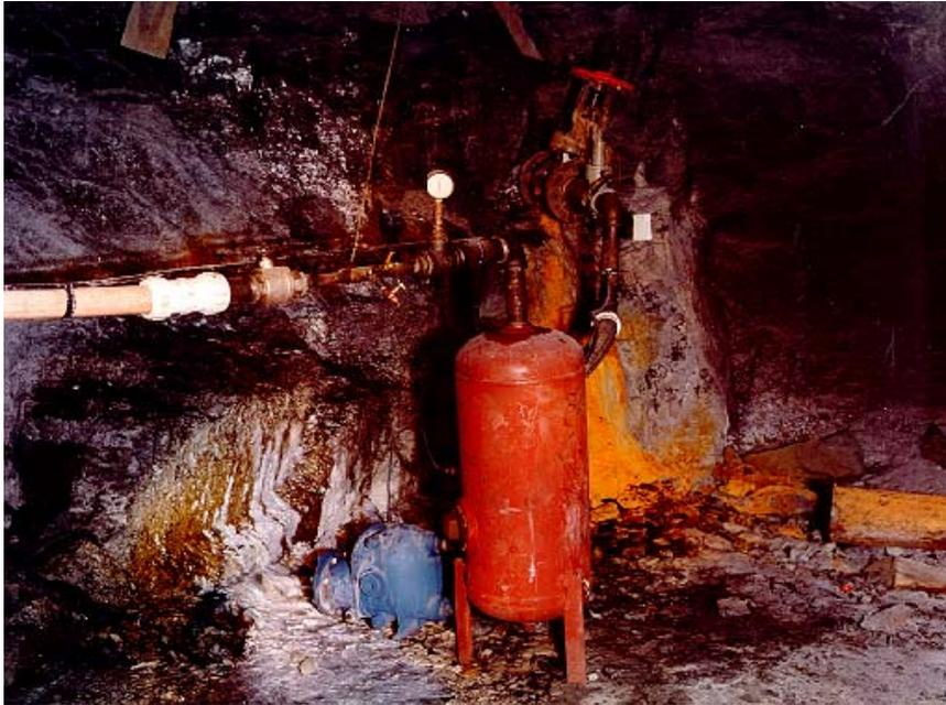
*Figure 6. Post drilling water separation and safety and monitoring system implemented by REI Drilling, Inc. at boreholes at the Soldier Canyon Mine.*
